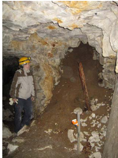
Maureen White (M.Sc., 2007) evaluating the collapse of overburden into a WWI tunnel at the Goodman subway tunnel.
